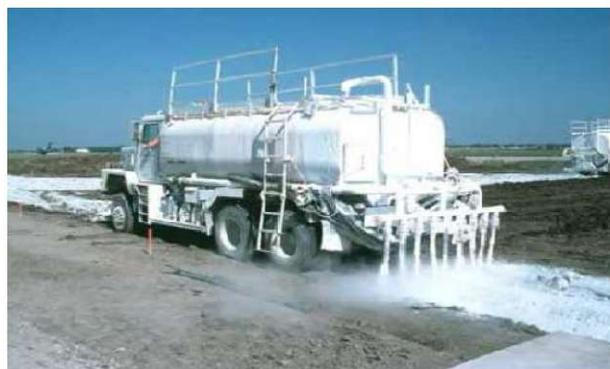
Figure 5. Sub-grade In-situ Lime Mixing Method
